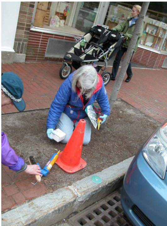
Carolyn Levy and Eileen Entin installing drain markers
